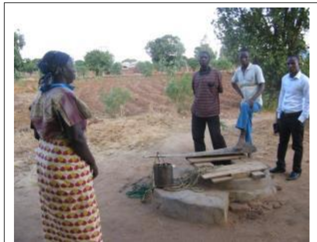
Fig 3.4 Traditional well with parapet, incomplete apron and cover, but no drainage channel.
