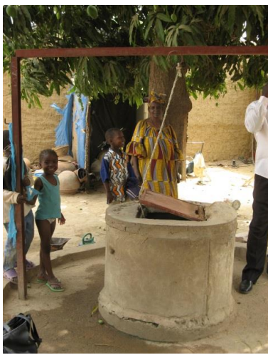
Fig 3.11. Rope stored on a post to keep it out of the dirt
