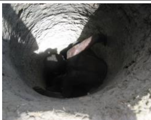
Fig 3.1 Njombwa well diggers tend to excavate at smaller diameters
