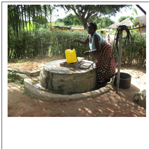
Fig 3.11. Rope stored on a post to keep it out of the dirt
