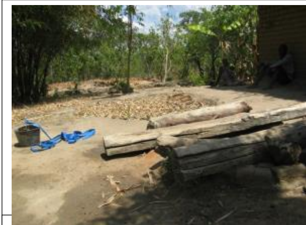
Fig 3.3 Family traditional well, with low parapet of mud bricks and timber to slightly reduce debris falling in and to make drawing water easier. (Njombwa)
